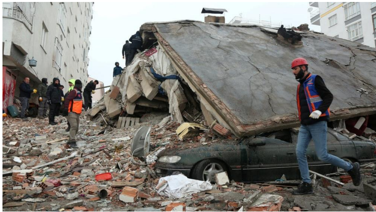
Figure 32. Collapsed structures, and rescue team searching for survivors in Diyarbakir city in Türkiye. Credit photo: Sertaç Kayar/Reuters
