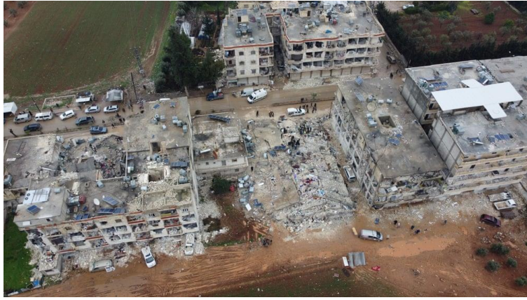
Figure 31. Collapsed building in in the Cenderes district of Aleppo, Syria. Credit photo: Anadolu Agency/Getty Images
