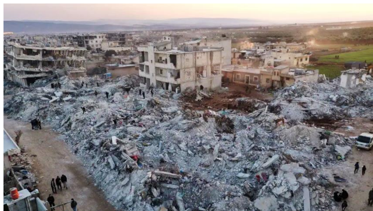
Figure 30. Completely collapsed buildings in the town of Jindires, Syria
