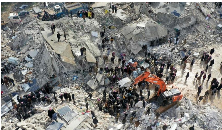
Figure 29. Collapsed building and rescue team searching for victims in the village of Besnia near the town of Harim, Idleb Governorate, Syria
