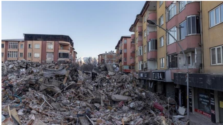
Figure 33. Collapsed structures in Elbistan, Türkiye. Credit photo: REUTERS/Maxim Shemeto
