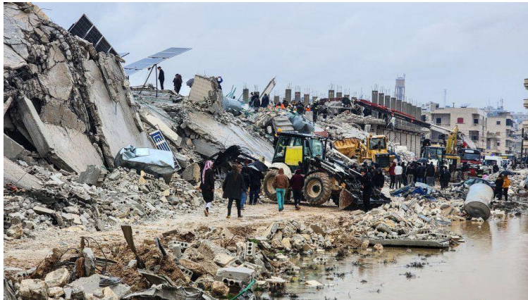
Figure 28. Collapsed building in Idleb region triggered by the M 7.8 Marash/Antep (Kehramanmarash) Earthquake as of 6 February 2023.
