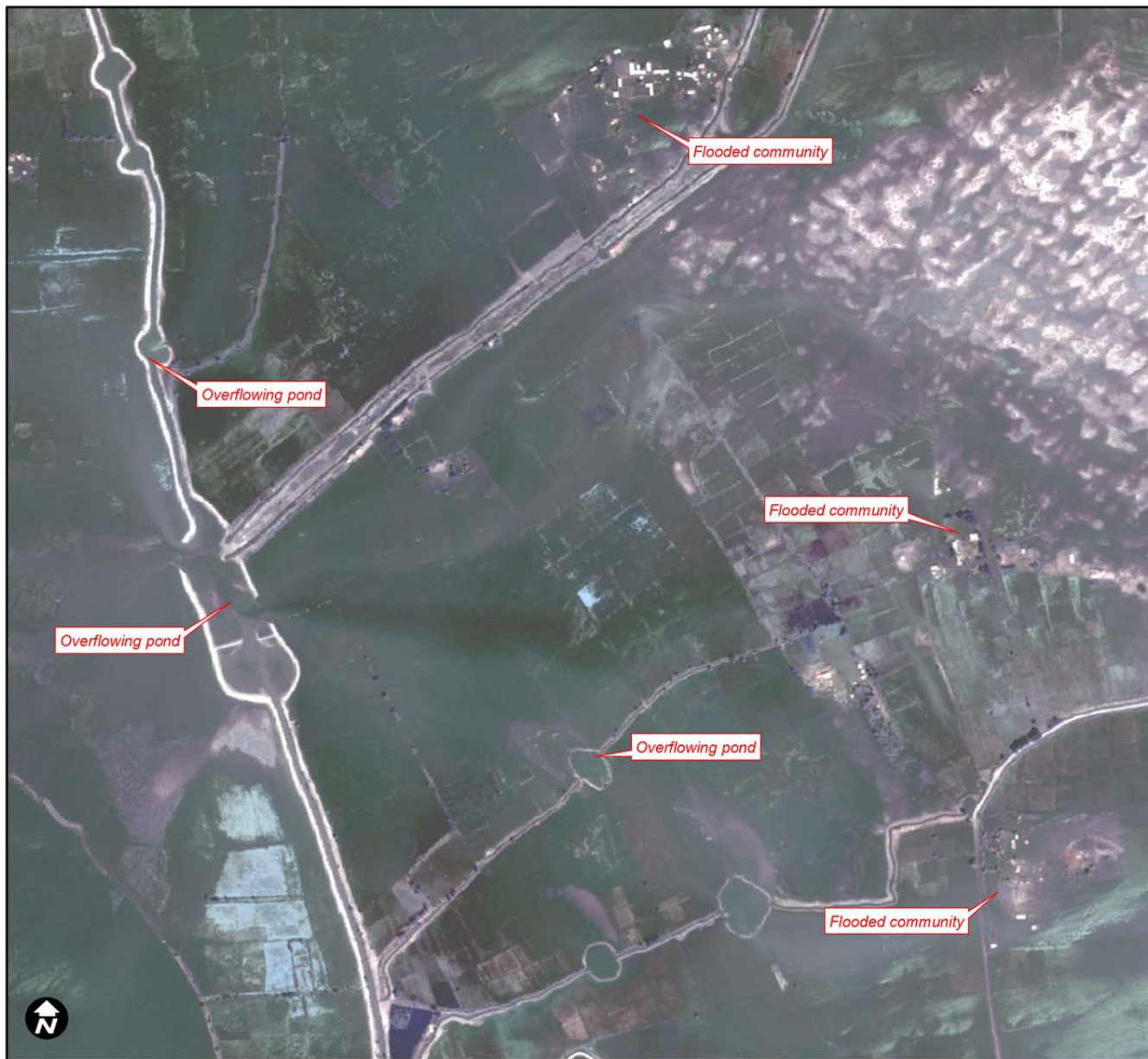
Site 4: Inundated agricultural land and overflowing ponds in a canal running east of the city.
