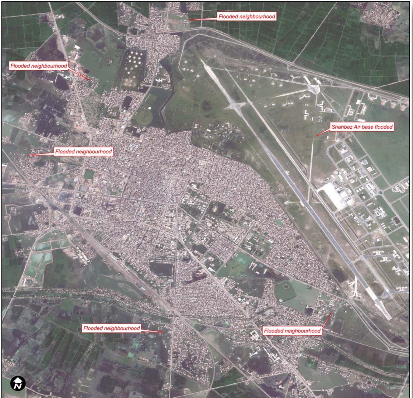
Site 2: Severe flooding of the Shahbaz Air Base and neighbourhoods on the outskirts of Jacobabad.
